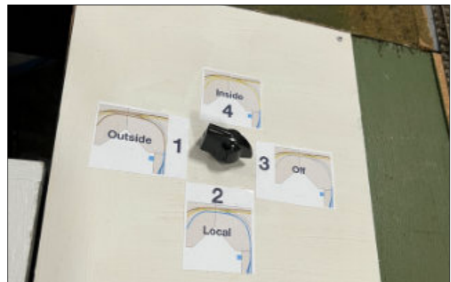
Figure 7: New Rotary Switch next to the blue yard throttle pack.
