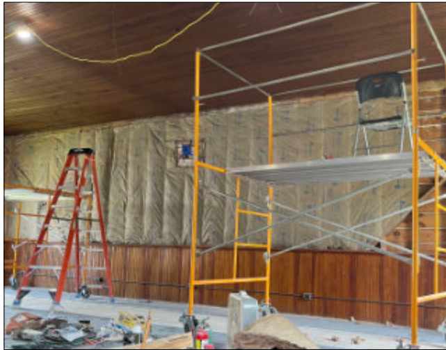
Figure 3: Fiberglass insulation is installed in the walls above the wainscot.
