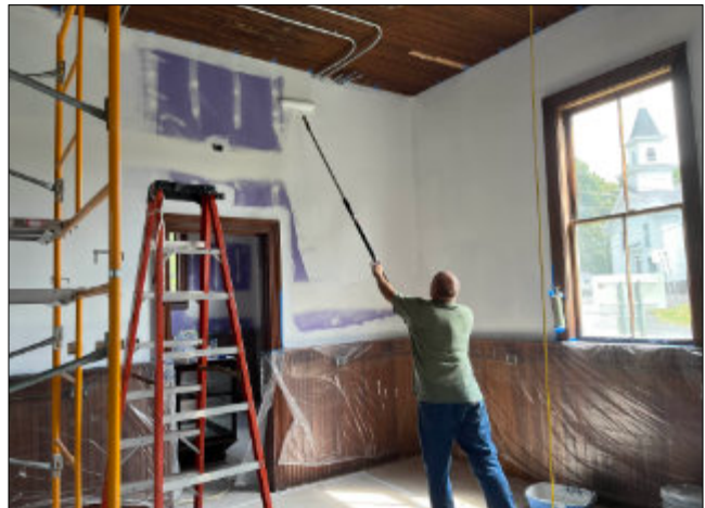
Figure 6: Shawn Connelly rolls on the primer coat of paint
