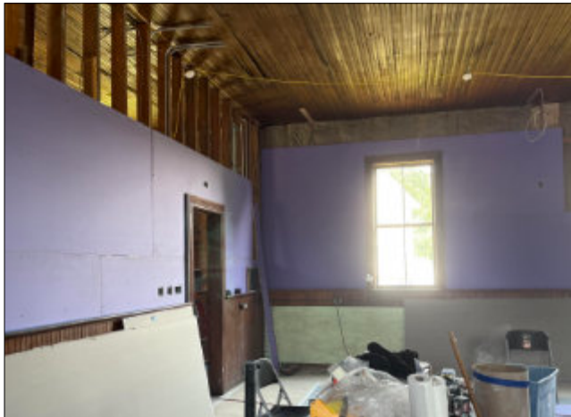
Figure 4: Drywall goes up
