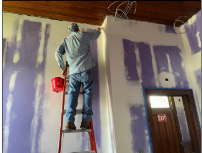
Figure 5: Todd Spencer working on “cutting in” with the primer paint
